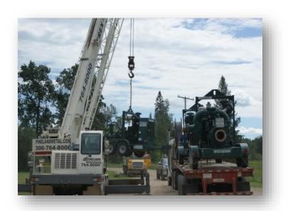
The City engaged a contractor to install a 6 kilometer line from the Little Red River to the sediment basins adjacent to the WTP. The Little Red water was pre-treated in the basins and pumped to the low lift pump house. Which was then treated through the WTP providing safe potable water. 8 Pumps were needed to move 22.5 million litres of water per day.
