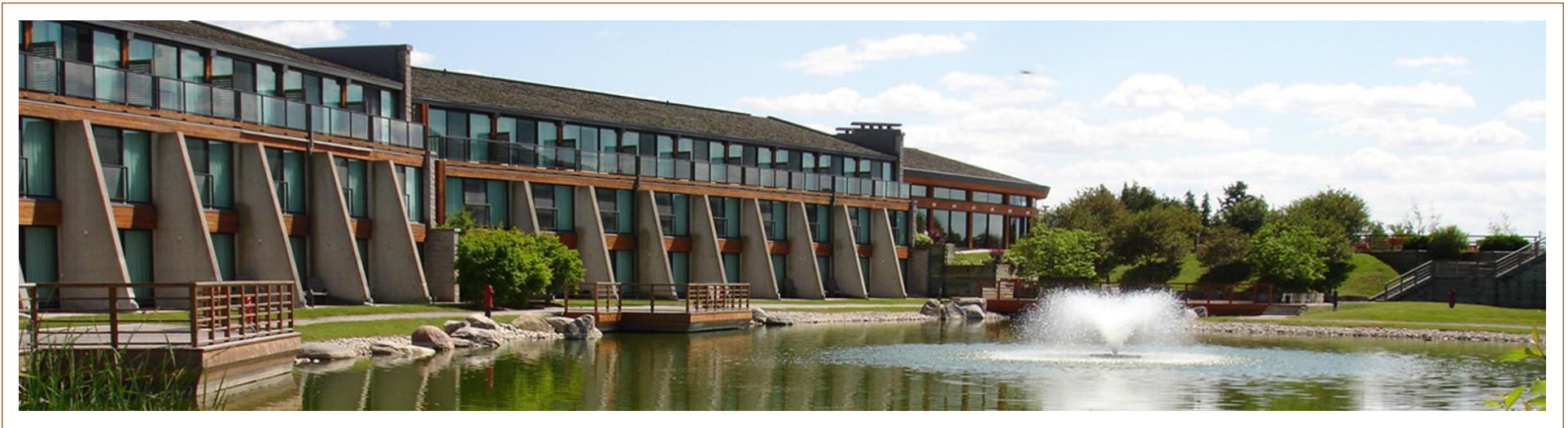
Kingbridge Centre, Toronto, Ontario
